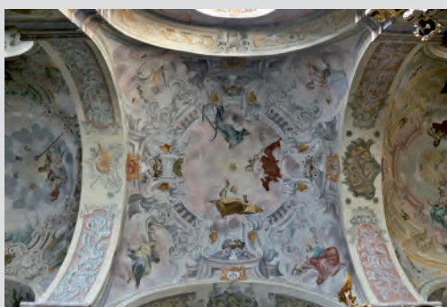
The polychrome of the aisle vault
