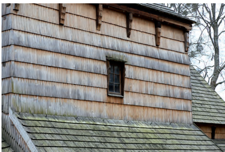
Orthodox church in Radruż – the northern wall of the nave
