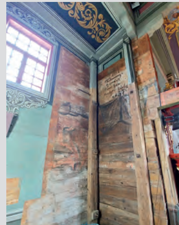
Gothic polychrome discovered on the walls in the north-eastern corner of the nave behind the altar of St. Barbara
